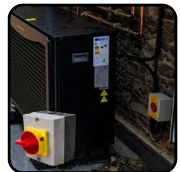
Rotary Isolator Switch
