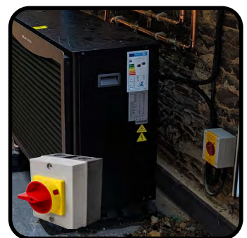
Rotary Isolator Switch
